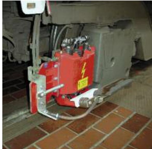
Carriage in a crane system
